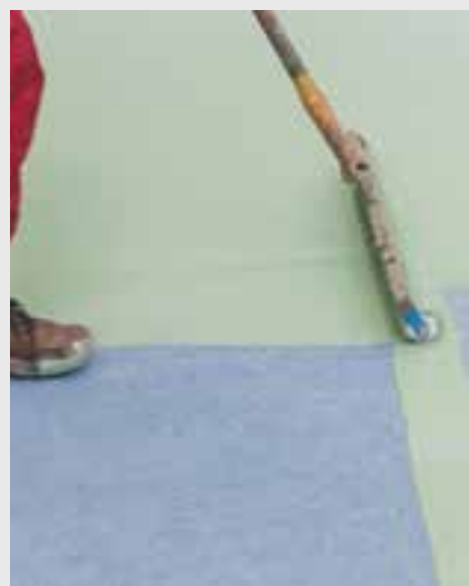
3 Apply the sealant by rolling it on with a velour roller
