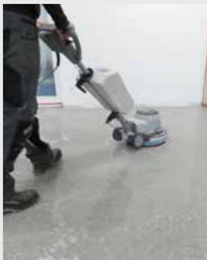
1 Cleaning the surfaces to be coated
