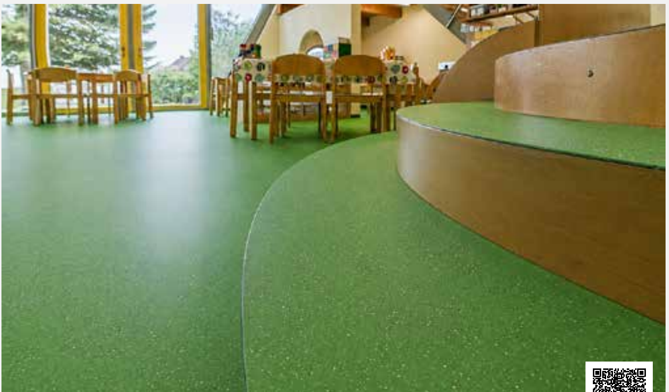
Afterwards: Seamless, coloured PU sealant with decorative chips embedded in it
