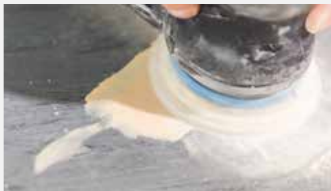
Grind the surface after hardening
