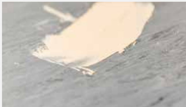
Filling with FLOOR SEALER 72 Repair
