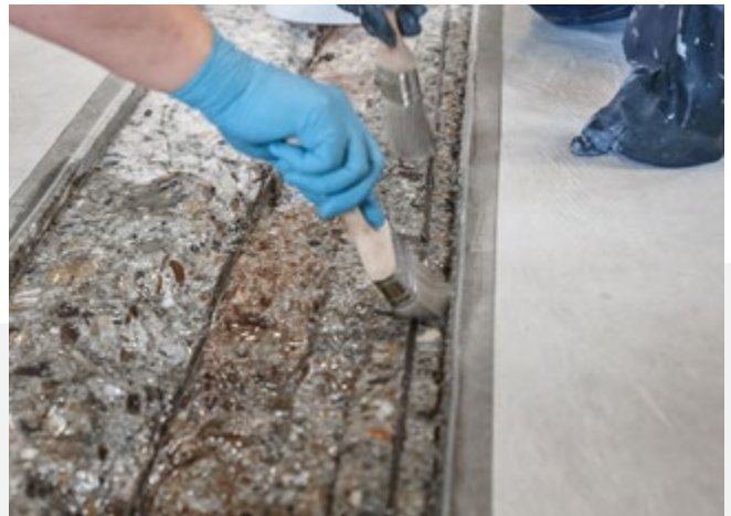
Priming the mortised joint area.
