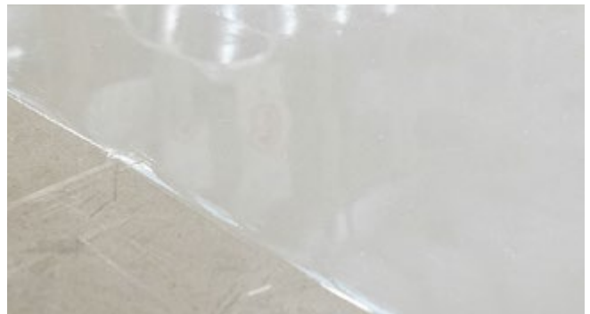
After: Joint grouting to floor level with KLB products.
