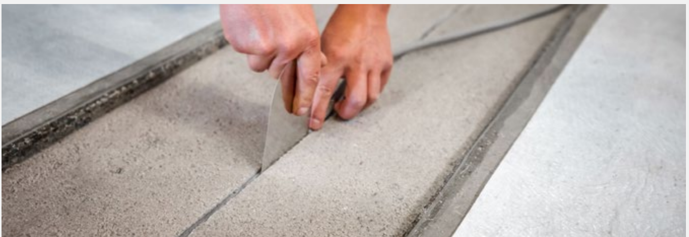
Insertion of the KLB PE round profile into the separating cut.
