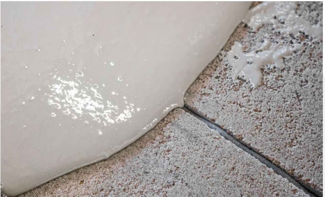
Good self-levelling properties make the grouting compounds easy to apply.
