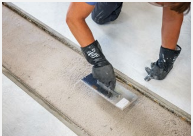
Use a fast-curing mortar for reprofiling to the required minimum layer thickness.
