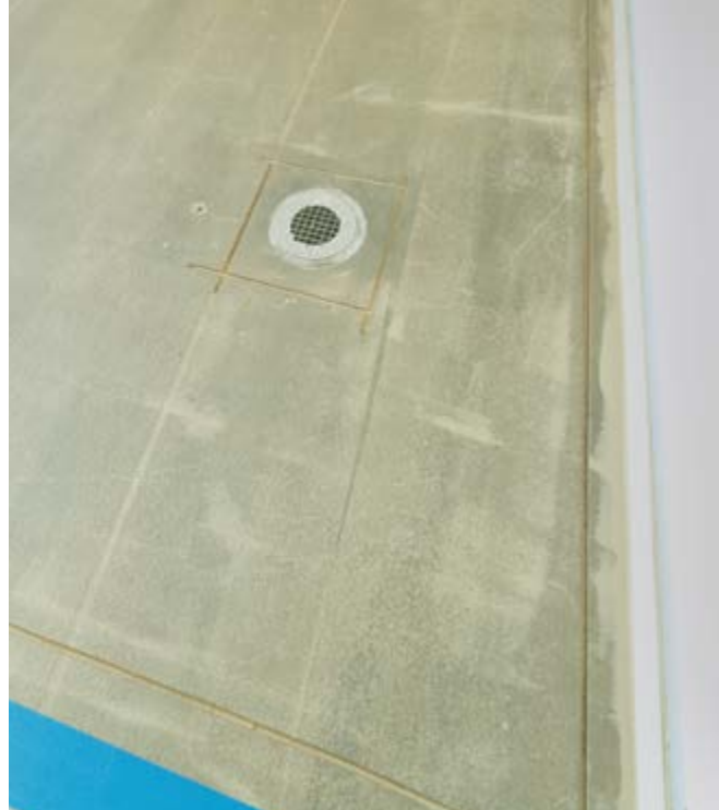
Cutting anchoring grooves during the installation of PU-BETON.
