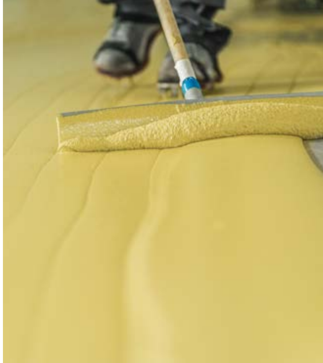
Higher layer thickness, particularly beneficial for areas exposed to heavy loads.
